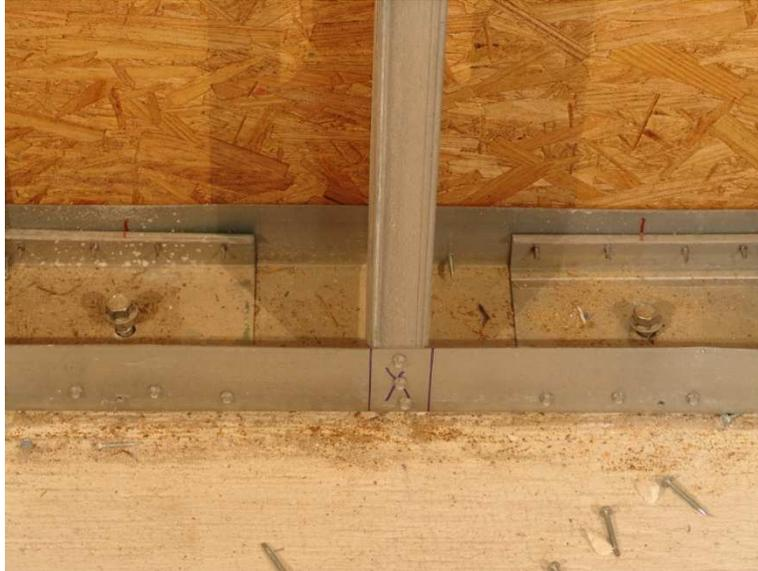
**Figure 1.** Conventional stud connection into a 7.62 cm (3") track with 3 screws.
