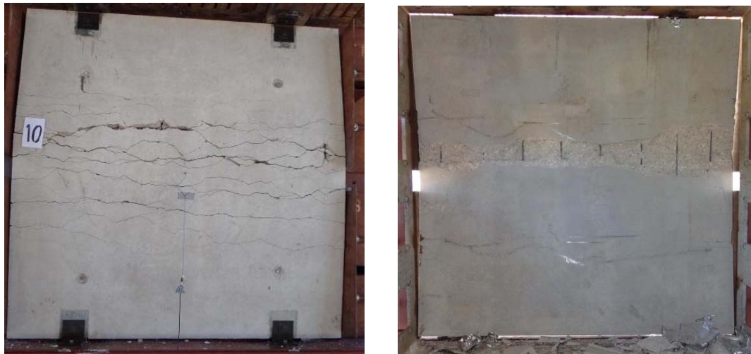
Figure 1. Exterior and Interior (Blast Loaded) Face of Test Panel with Heavy Damage
