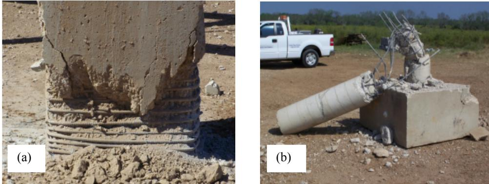
**Figure 1.** (a) Column Spall (b) Column Breach
