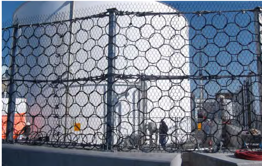
Figure 7. Photograph of Installed Perforated Barrier
