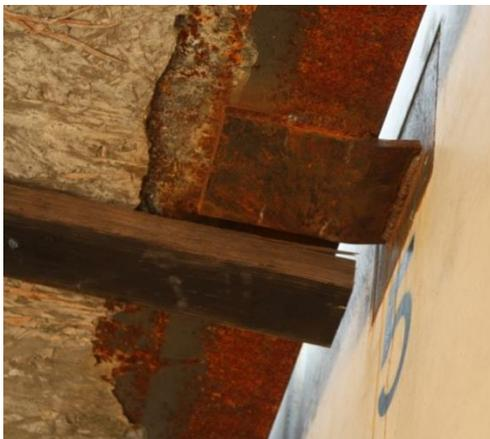
*Upward panel movement acting on weld*
